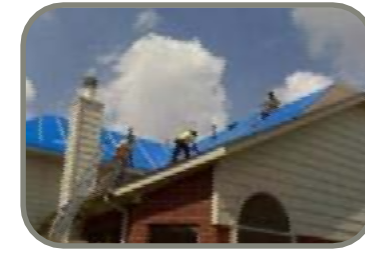
Temporary Roofing “Blue Roofs”
